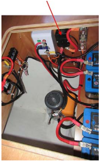
Control panel for electrically controlled battery breakers
