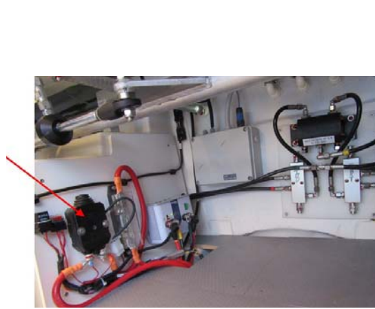
Positive isolator switch (Bow thruster)
